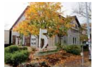
⑮ OLD FIRESTATION BUILDING
