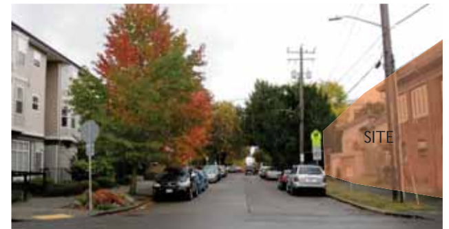
② LOOKING SOUTH UP INTERLAKE AVENUE N
