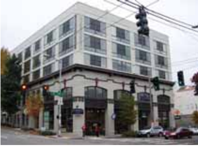
PACKARD BUILDING,, CAPITOL HILL
